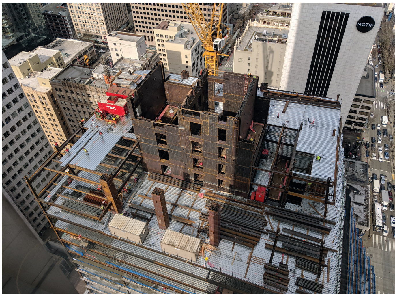
Fig. 2 — Rainier Square Tower erection using the SpeedCore system. (Photo courtesy of Magnusson Klemencic Associates.)
