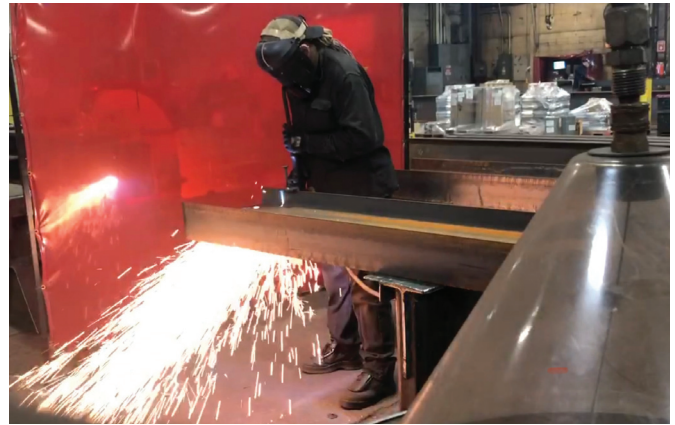
Tonya Robarge works at LeJeune Steel Co., where she is employed as a welder/fabricator.
