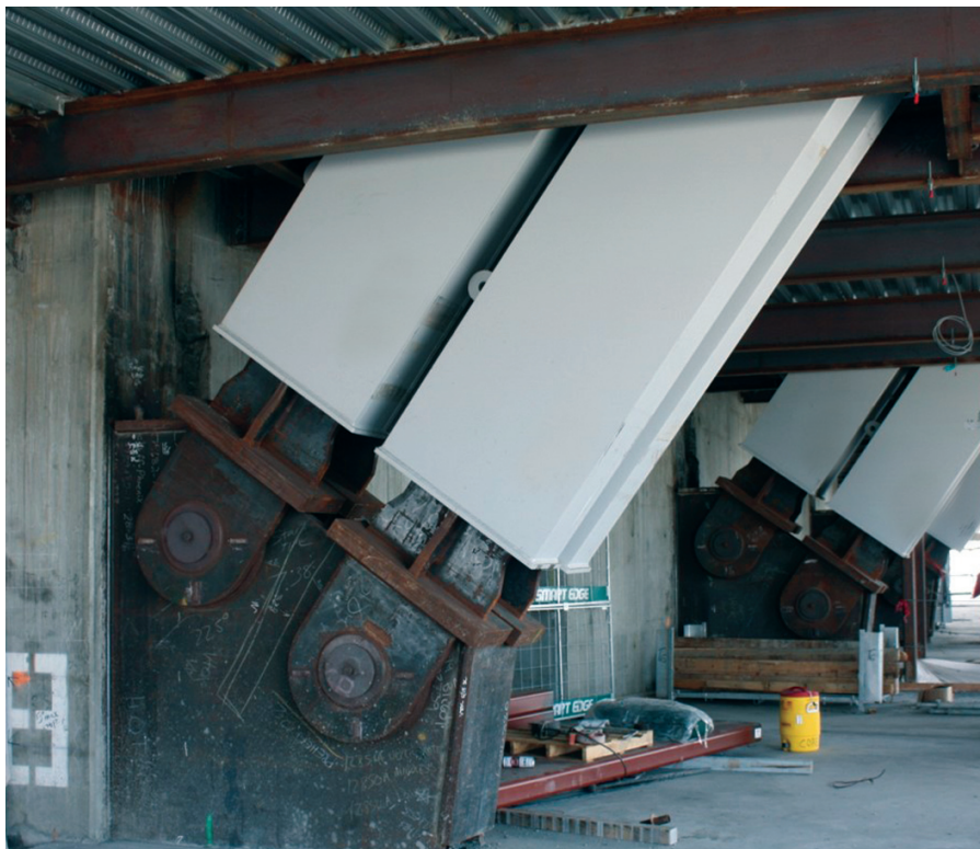
Fig. 1 — ESW-NG process application at the Wilshire Grand Hotel, Los Angeles, Calif. (Photo courtesy of Schuff Steel Co.)
