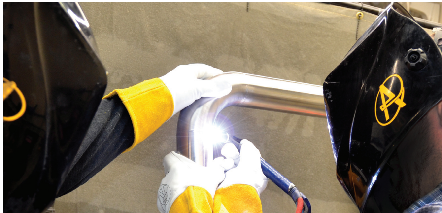
Fig. 3 — Welder Tom Hammer assists Welder Brian Thessen as he performs GTAW on a large stainless steel tube. The art of GTAW produces exceptionally high-quality, refined, and superior welds.
